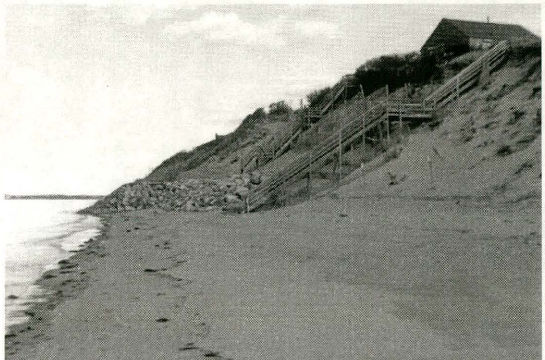
Revetment construction on an eroding coastal bank in Eastham, MA, has resulted in the loss of the coastal beach fronting the structure.
