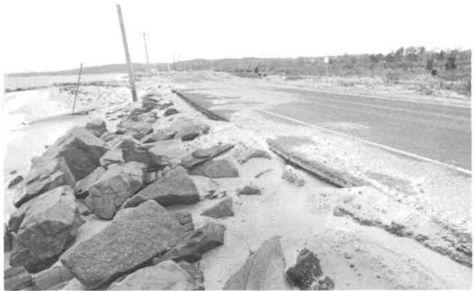
*Undercutting was also apparent, to a lesser degree, along the straightway of Surf Drive between the beach houses and Elm Road.*
