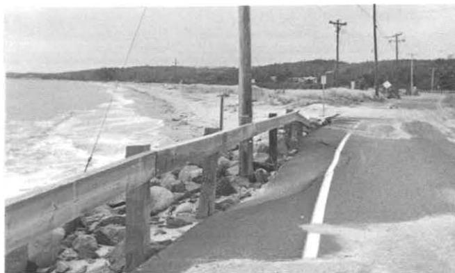
*Undercutting of the road was most apparent in the area of Surf Drive that is intersected by the Shining Sea Bikeway, near Oyster Pond Road. In one area, the undercutting caused the road to collapse, as the sand supporting the asphalt was washed out to sea.*
