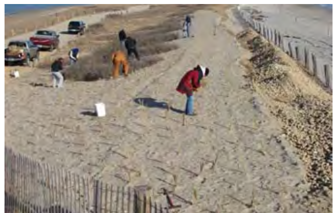
Figure 4. Planting the artificial dune with beachgrass.
