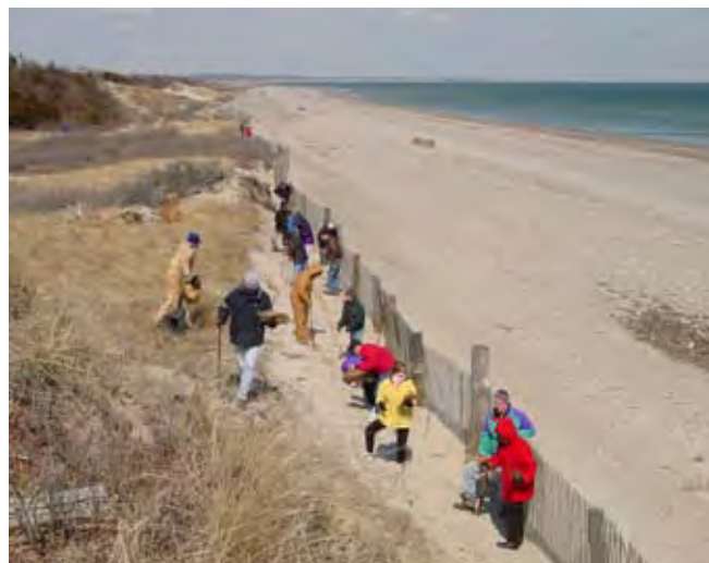
Figure 21. Planting foredune scarps is particularly important.
