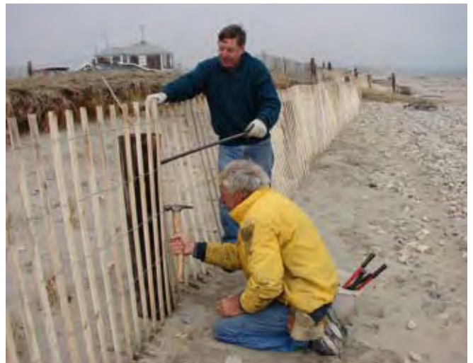
Figure 13. Experienced sand fence installers Joe Grady and Dick Sjostedt attach fencing to posts. The snow fence is being held taut by a crow bar while a 2" galvanized staple is hammered into the post loosely attaching the snow fence 'wire' to the post.
