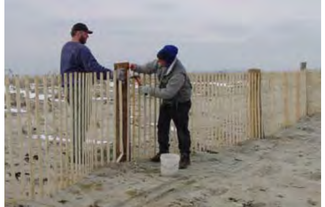
Figure 12. Fence is attached to 6" diameter posts.
