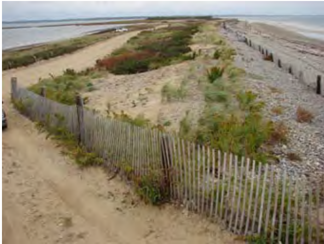
Figure 5. Artificially built dune naturally revegetating.
