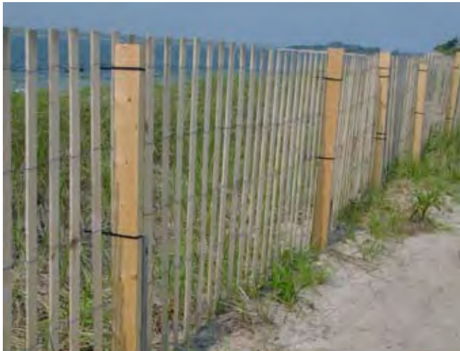
Figure 15. Sand/snow fence held to 2x4 posts with tie-wraps, an alternate method of installation.
