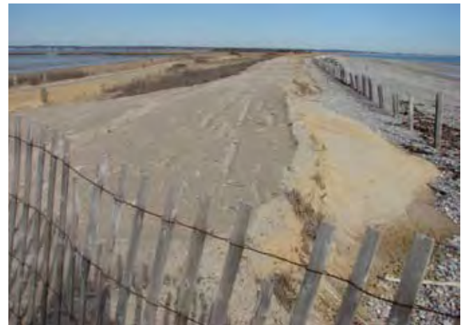
Figure 3. Covering quarry sand with natural dune sand.
