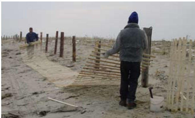
Figure 11. Fence is laid-out.
