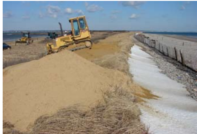
Figure 2. Building a dune with imported quarry sand (Duxbury Beach, Mass.).
