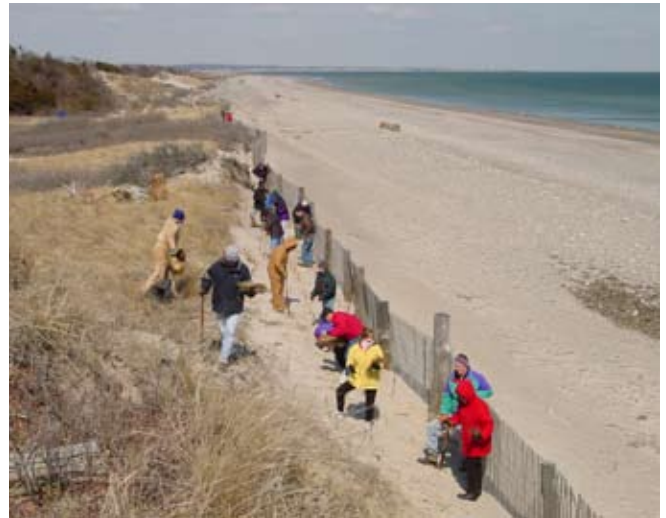
Figure 21. Planting foredune scarps is particularly important.
