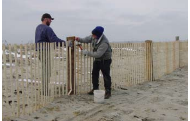
Figure 12. Fence is attached to 6" diameter posts.
