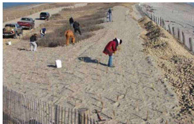
Figure 4. Planting the artificial dune with beachgrass.
