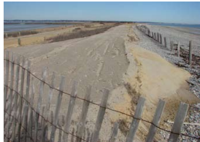
Figure 3. Covering quarry sand with natural dune sand.
