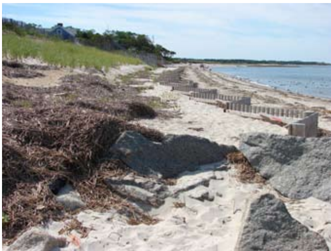
Figure 6. An artificial dune 18 months after construction.
