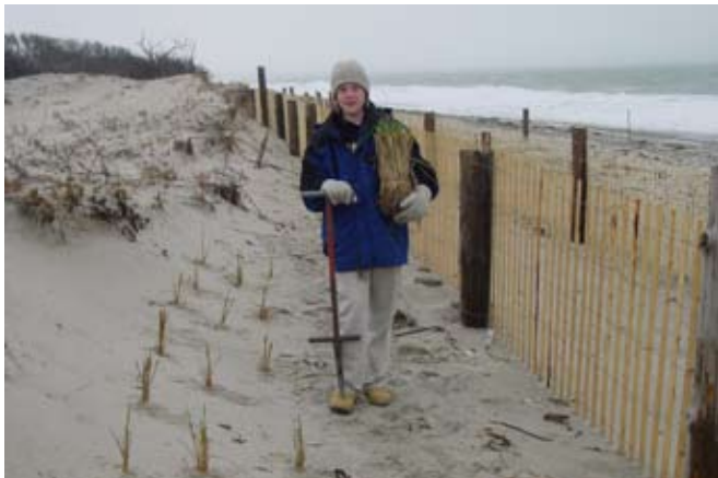
Figure 19. Planting ‘Cape’ American beachgrass requires only a pogo-type hole poker (any pole or stick several feet long will do), and culms of beach grass (100 culms in a bundle as shown). Note the horizontal bar on the pogo stick is approximately 8” inches up from the bottom for ease of ensuing proper depth of the hole. Makai O’Connell planting beachgrass on Duxbury Beach, Mass.
