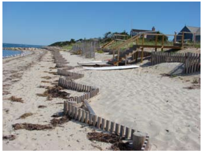
Figure 18. Double row of sturdy sand drift fence — made of 2x3 vertical and horizontal rows with 6" diameter posts which are partially buried when installed. This style of fence is generally used in areas of small waves or ice.
