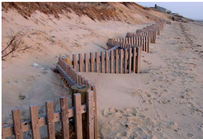
Figure 17. Sturdy sand drift fence made of 2x3 vertical and horizontal members, with 6" diameter posts.
