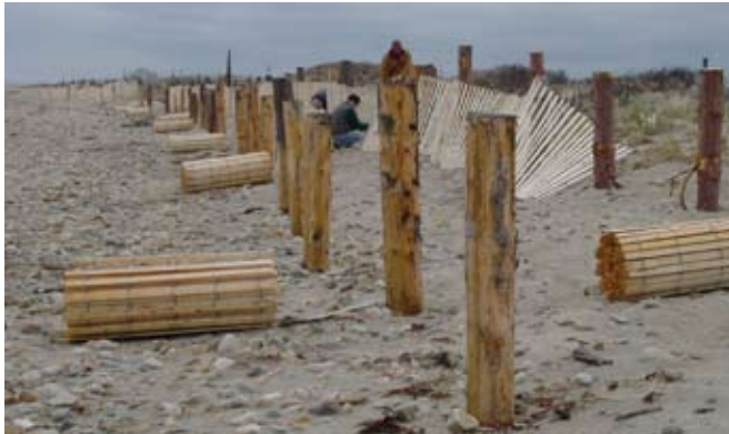
Figure 10. Installing 6" piles for a double row of slat style fence.
