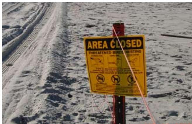
Figure 23. Preserve piping plover habitat and areas for pioneer beach and dune vegetation growth fronting the foredune by roping off the area.
