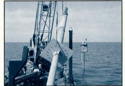
Supported by Sea Grant and the U.S. Coast Guard, University of New Hampshire engineers Ken Baldwin, Pedro de Alba, and Rob Swift, left to right, developed a pile designed to mark navigational channels and survive collisions with tugs and barges. To the left, the researchers study a scale model; above, a Coast Guard crew installs one of the devices in the Houston Ship Channel.
