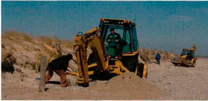
Figure 8. Using an excavator to dig larger size holes for 6" to 8" poles, Duxbury Beach, Mass.
