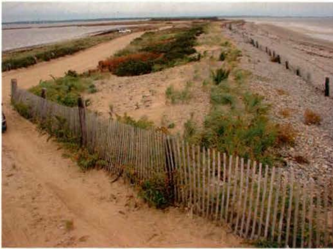
Figure 5. Artificially built dune naturally revegetating.
