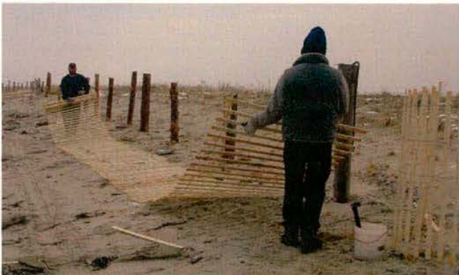
Figure 11. Fence is laid-out.
