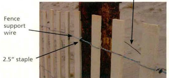
Figure 14. A wire is wrapped around the back of the post and is attached to the sand fence wire approximately 8" to either side. This adds support to the fence under strong wind conditions. A loose attachment allows the fence wire to slide and move to prevent breakage as wind shakes the fence.
