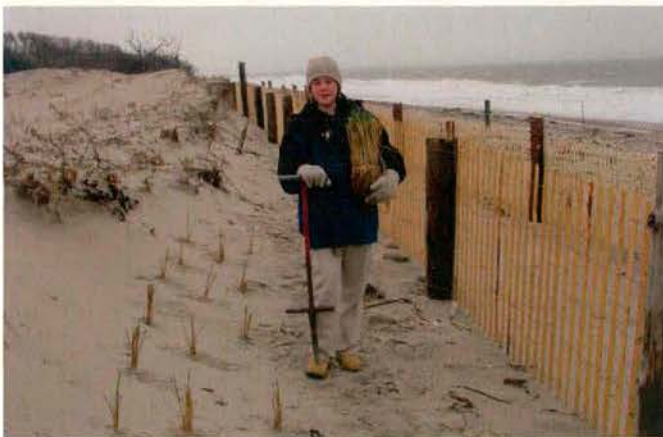
Figure 19. Planting 'Cape' American beachgrass requires only a pogo-type hole poker (any pole or stick several feet long will do), and culms of beach grass (100 culms in a bundle as shown). Note the horizontal bar on the pogo stick is approximately 8" inches up from the bottom for ease of ensuring proper depth of the hole. Makai O'Connell planting beachgrass on Duxbury Beach, Mass.
