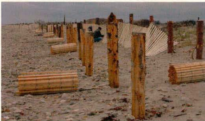
Figure 10. Installing 6" piles for a double row of slat style fence.
