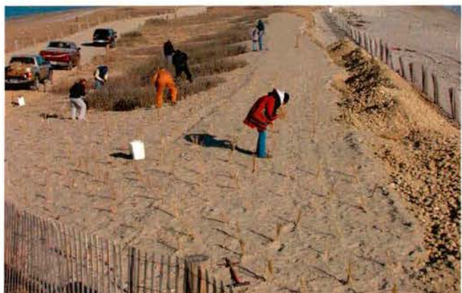
Figure 4. Planting the artificial dune with beachgrass.
