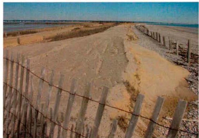
Figure 3. Covering quarry sand with natural dune sand.
