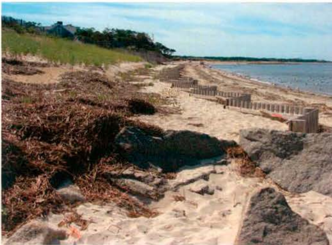
Figure 6. An artificial dune 18 months after construction.
