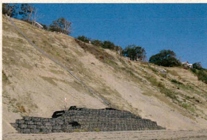
Preventing a sand source from eroding, as shown here, will cause accelerated erosion of the shoreline.
