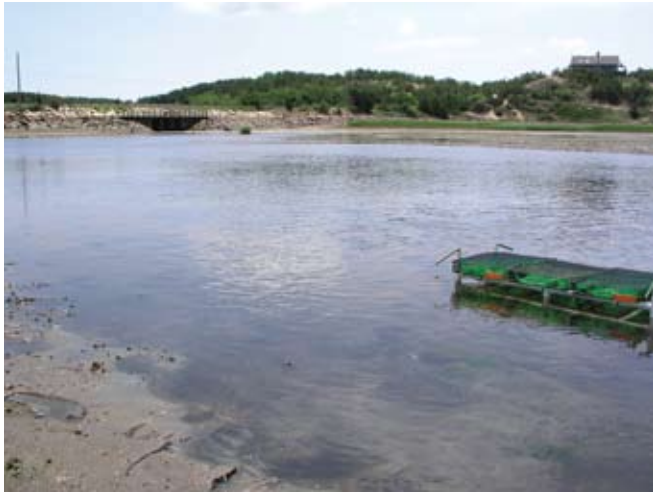
Many communities have opted to restore tidal flow by opening tide gates in dikes such as this one in the Herring River, Wellfleet, Massachusetts.
