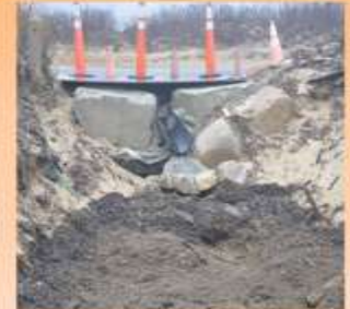
Culvert damage from Sandy, awaiting FEMA repairs, further compromised during January 2014 Nor'easter
