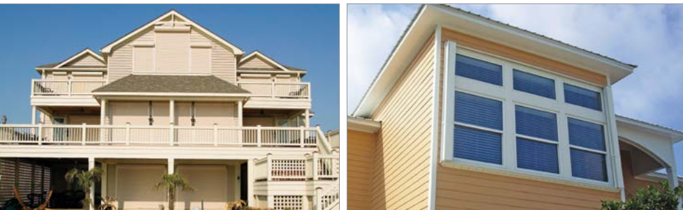
Figure 4-9. Coastal home protected with roll-down shutters on all windows and doors. The shutter is held in place by vertical guide tracks and can be deployed manually or with an integrated electric motor. Image courtesy of QMI, Inc.
