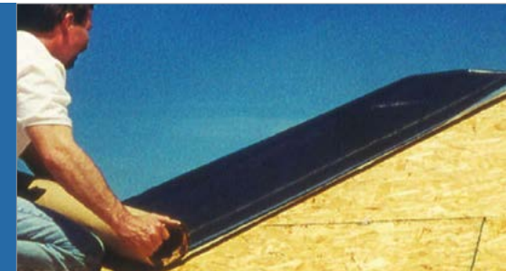
Figure 4-8. Synthetic underlayments are typically made from polypropylene, polyester, or fiberglass fabric, which weighs less than felt building paper, can be manufactured with anti-slip surfaces, and can withstand exposure to the elements for six months. Image courtesy of Carlisle Coatings & Waterproofing.
