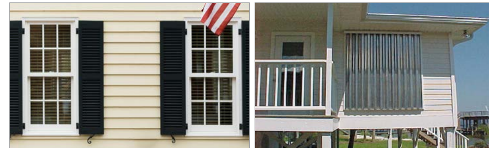
Figure 4-11. Colonial shutters that are suitable for storm protection are typically made of aluminum or fiberglass. During a storm, the panels are closed and secured along the vertical center of the window. During good weather, the panels open along hinges on the side of the window and rest flat against the wall in a decorative manner.
