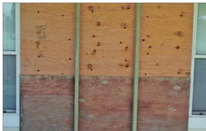
Figures 4-16 and 4-17. Not only is it necessary to install plywood opening covers correctly, it is also important to correctly label them and store them away from heat and humidity. Images courtesy of Dennis Hwang.
