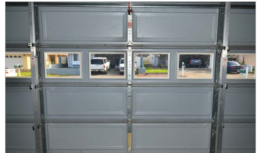
Figure 4-20. Vertical braces such as these can be deployed during high-wind events to strengthen the garage door. The braces are secured from the header over the garage door to the fasteners installed in the concrete floor. Deployment and breakdown are about 10 minutes each. The windows have been covered with a laminate film. Image courtesy of Dennis Hwang.
