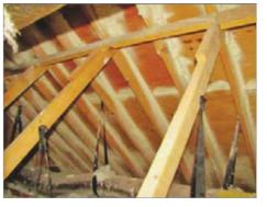
Figure 4-5. Spray polyurethane foam is used to add strength between the rafters and the plywood sheathing. This method can be used to strengthen existing roofs and may negate the need to replace older roofs. It can also be used where fasteners are missing or at the corners of hip style roofs or the ends of gable end roofs, which are especially susceptible to wind forces. See FEMA publication numbers P-499 and P-804. Image courtesy of
