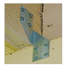
transferred to the horizontal floor or roof system, using the shear strength in the floor or roof to resist the applied wind load. This is now required in new construction near an open field or on the water with few other structures or trees to break up the wind.
