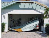
because the door is closing against the door jamb, which provides resistance to the door being pushed in by high winds.
