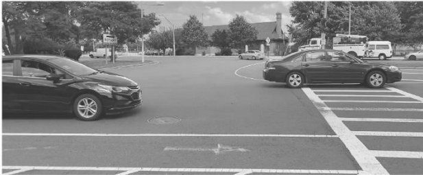
BARRIERS UNSAFE CROSSINGS + BARRIER TO WATER
