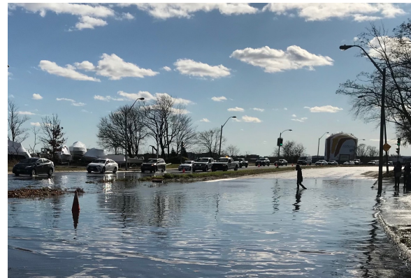
Morrisset Blvd, Boston, High-Tide Flooding (Streetsblog.org)
