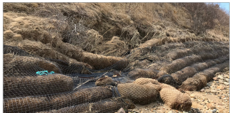
If a biodegradable stabilization method does not maintain proper sand cover it will deteriorate much more quickly than the design life of the array.
