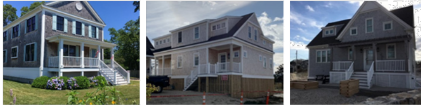
A traditional one-story porch (left) helps reduce the apparent size of the building behind it. Inset porches (center and right) create a space that breaks up a larger building mass.
