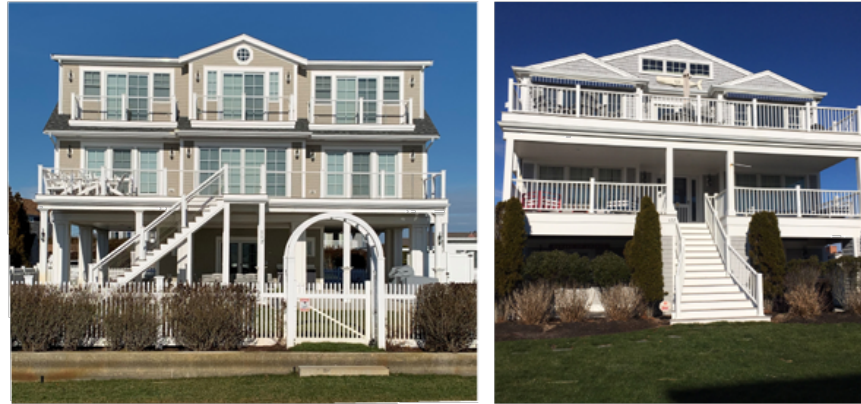
These elevated buildings maintain open patios beneath and incorporate landscaping at the building edge and the streetscape edge to provide some pedestrian scale.
