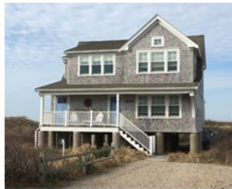
Open spaces under porches, ells, or the entire structure help to reduce the overall scale of an elevated building.
