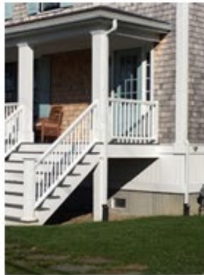
Open spaces under porches, ells, or the entire structure help to reduce the overall scale of an elevated building.
