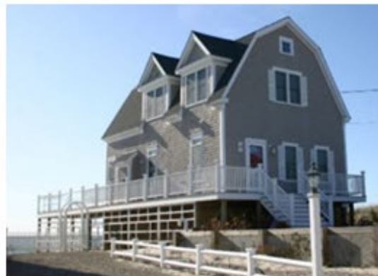
Architectural detailing with lots of space between elements can define the area under a deck without blocking views through the space.
