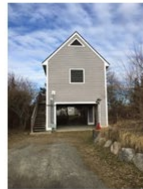
Open spaces under porches, ells, or the entire structure help to reduce the overall scale of an elevated building.
