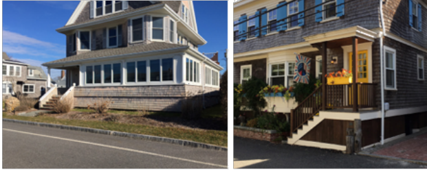
Left: Falmouth home with extended stairs that face the street and keep the entry prominent. Right: Provincetown home with stairs turned 90 degrees due to narrow setback from street.
