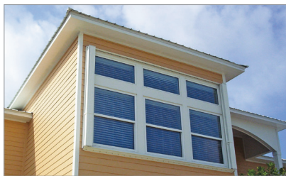
Figure 3-10. Accordion shutter (shown in the open position) installed over a large window of a coastal home. Shutter has been installed to allow deployment from inside the home. Image courtesy of Roll-a-way.
