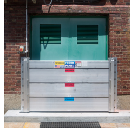
Figure 3-18. Image of dry floodproofing courtesy of ResilientWoodsHole
