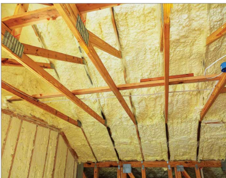
Figure 3-5. Spray polyurethane foam is used to add strength between the rafters and the plywood sheathing. This method can be used to strengthen existing roofs and may negate the need to replace older roofs. It can also be used where fasteners are missing or at the corners of hip style roofs or the ends of gable end roofs, which are especially susceptible to wind forces. See FEMA publication numbers P-499 and P-804. Image courtesy of FEMA.
