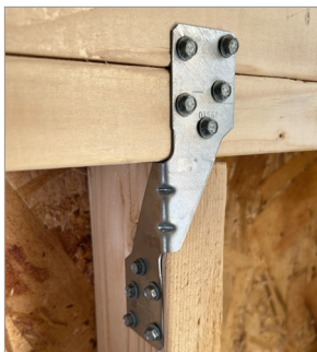
Figure 3-6. This is an example of retrofitting an existing house originally built without hurricane clips. The popular H3 clip is used here; four nails attach the clip to the roof (truss-rafter) and four more nails attach to the wall or top plate below. For a retrofit, the clips are exposed on the outside of the house; therefore, both the clip and fasteners should be corrosion-resistant and painted to blend with the exterior of the house. With the correct clip and nails, you could perform the work or, if you prefer, hire a licensed contractor. Photo credit: WHOI Sea Grant.
