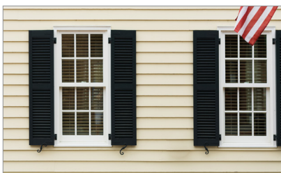
Figure 3-11. Colonial shutters that are suitable for storm protection are typically made of aluminum or fiberglass. During a storm, the panels are closed and secured along the vertical center of the window. During good weather, the panels open along hinges on the side of the window and rest flat against the wall in a decorative manner.
