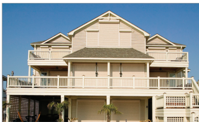
Figure 3-9. Coastal home protected with roll-down shutters on all windows and doors. The shutter is held in place by vertical guide tracks and can be deployed manually or with an integrated electric motor. Image courtesy of QMI, Inc.
