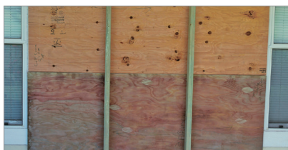
Figures 3-14 and 3-15. Not only is it necessary to install plywood opening covers correctly, it is also important to correctly label them and store them away from heat and humidity. Images courtesy of Dennis Hwang.
