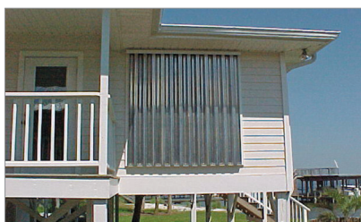
Figure 3-12. These 0.050 gauge aluminum storm panels offer cost effective storm protection. In this example, panels slip into a track above the window and secure onto a bottom track using wing nuts. Image courtesy of Roll-a-way.
